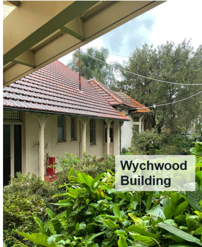
South elevation of Wych Wood Building
