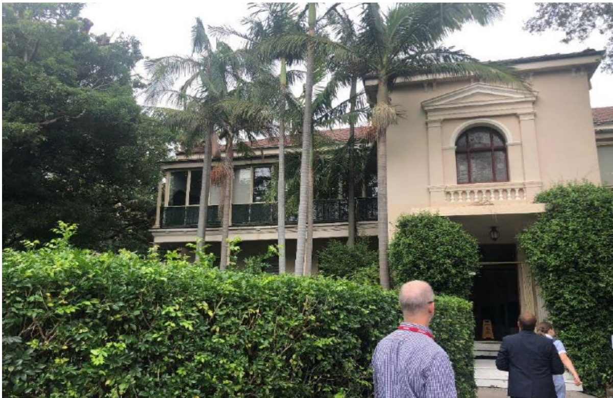
east elevation of Administration Building
